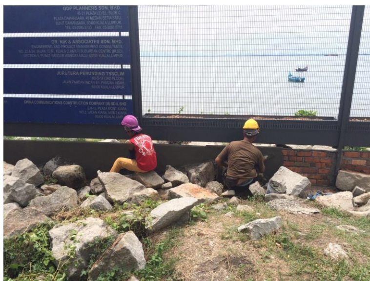
(Above) Ongoing construction of the low brick wall.
