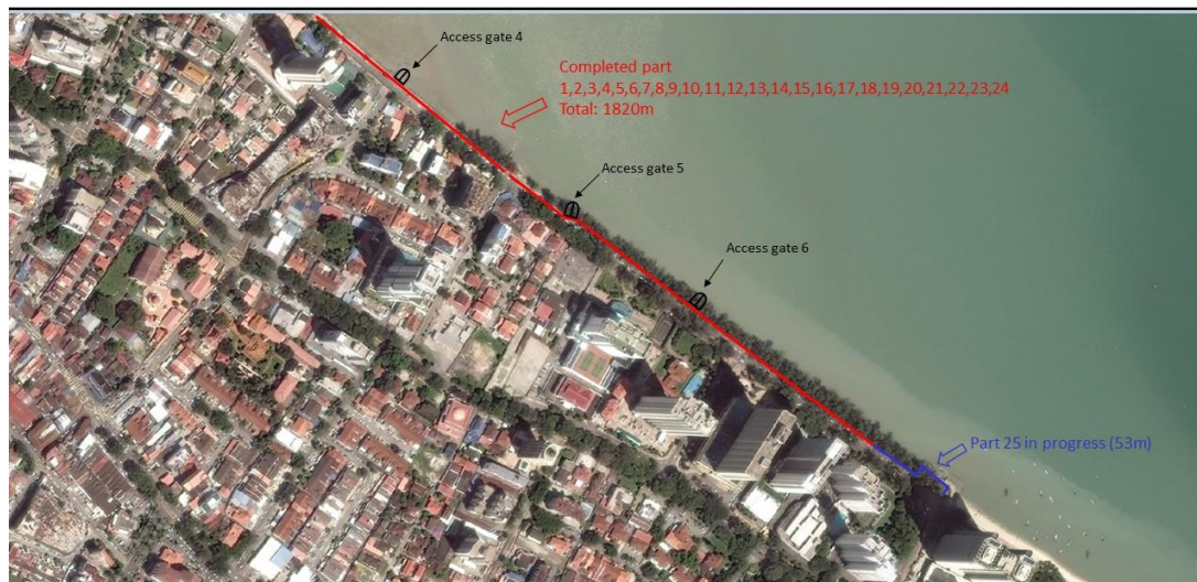
Aerial view of fencing works progress
