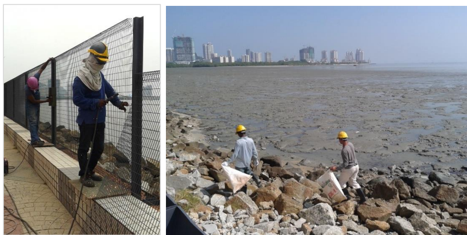
(Left) Mesh fencing being installed along Gurney Drive; (right) Workers cleaning up the shore area near the fencing
