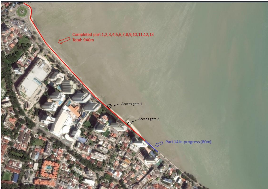
Aerial view of fencing works progress
