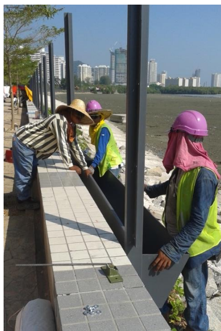
Mounting up planter boxes (left); Installing mesh fencing material (right)
