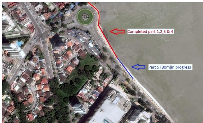
Aerial view of fencing works progress
