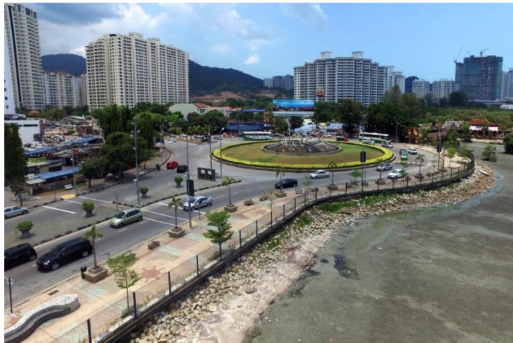
View of the completed permeable fencing from the sea
