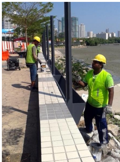
Workers painting the metal structures
