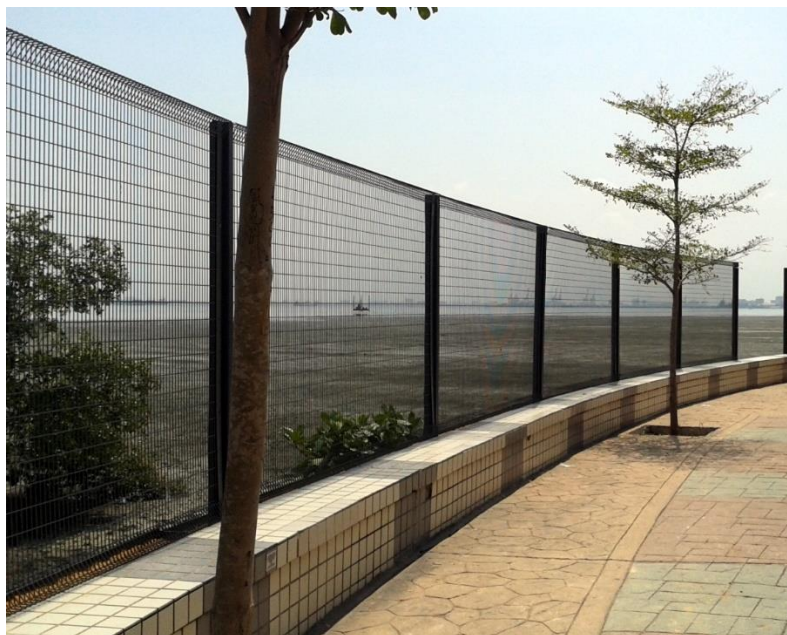
Completed section of mesh fencing
