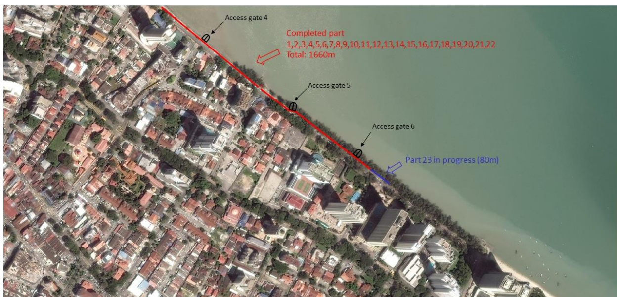
Aerial view of fencing works progress
