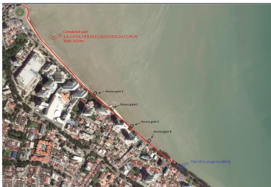
Aerial view of fencing works progress
