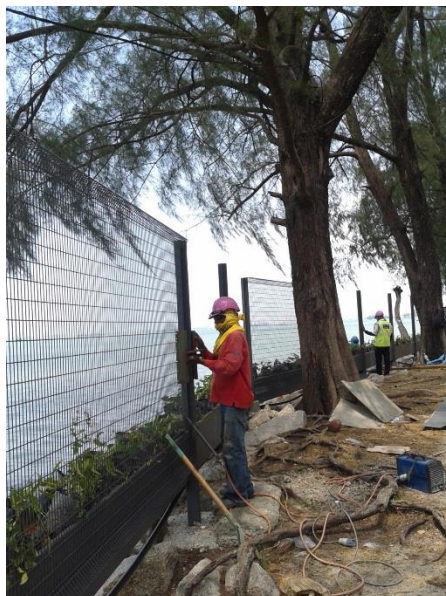
(Above) Workers installing fencing poles at the latest 80-m stretch.
